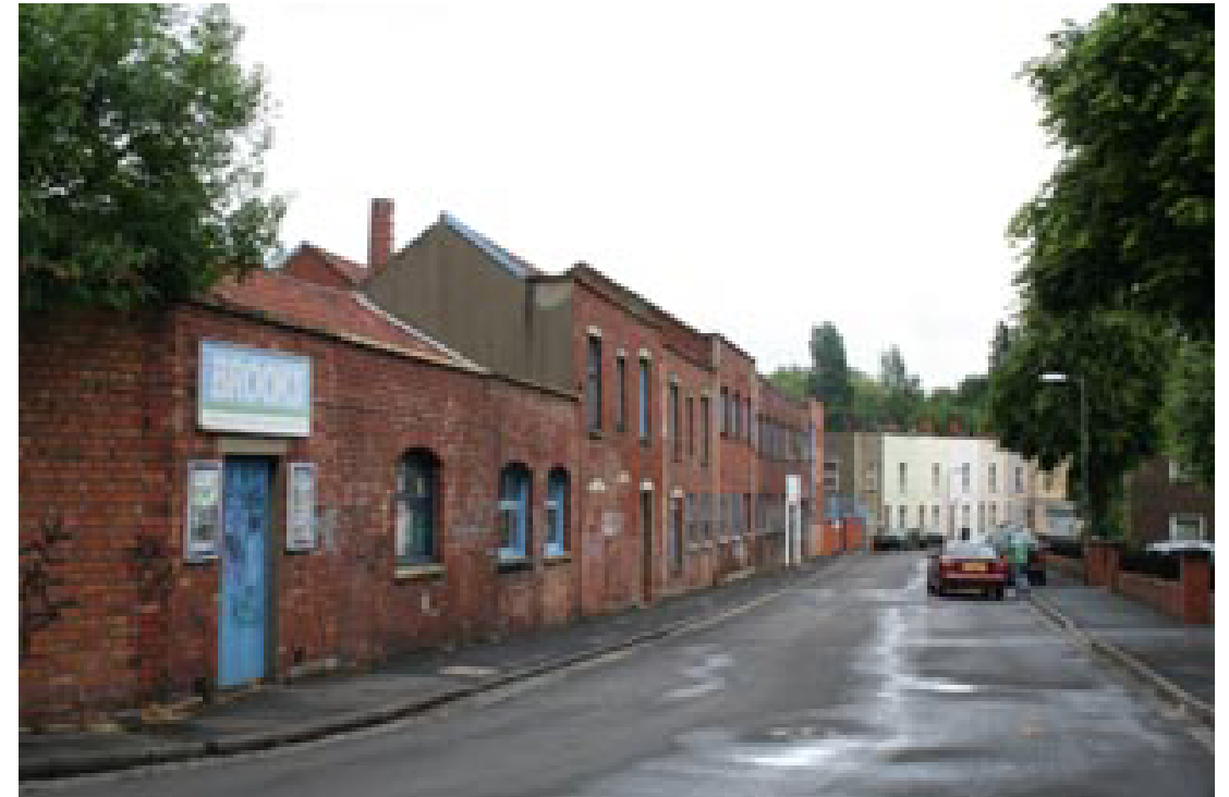
Morley St brick built workshops
